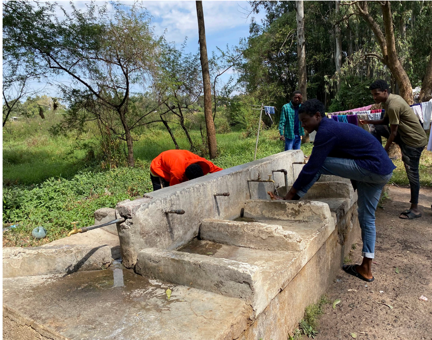
Multipurpose Outdoor Faucets
